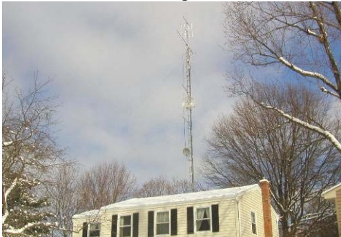
Here is an old picture of the tower and antennas before we started dismantling it.
